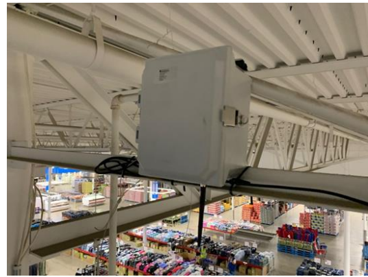
SeniMax™ Gateway at roof system of a building/warehouse for data acquisition
