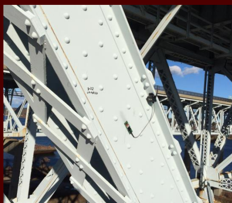
Resensys SenSpot™ sensors monitor 6000 -foot Gold Star Memorial Bridge (I-95 over Thomas River, Connecticut)
