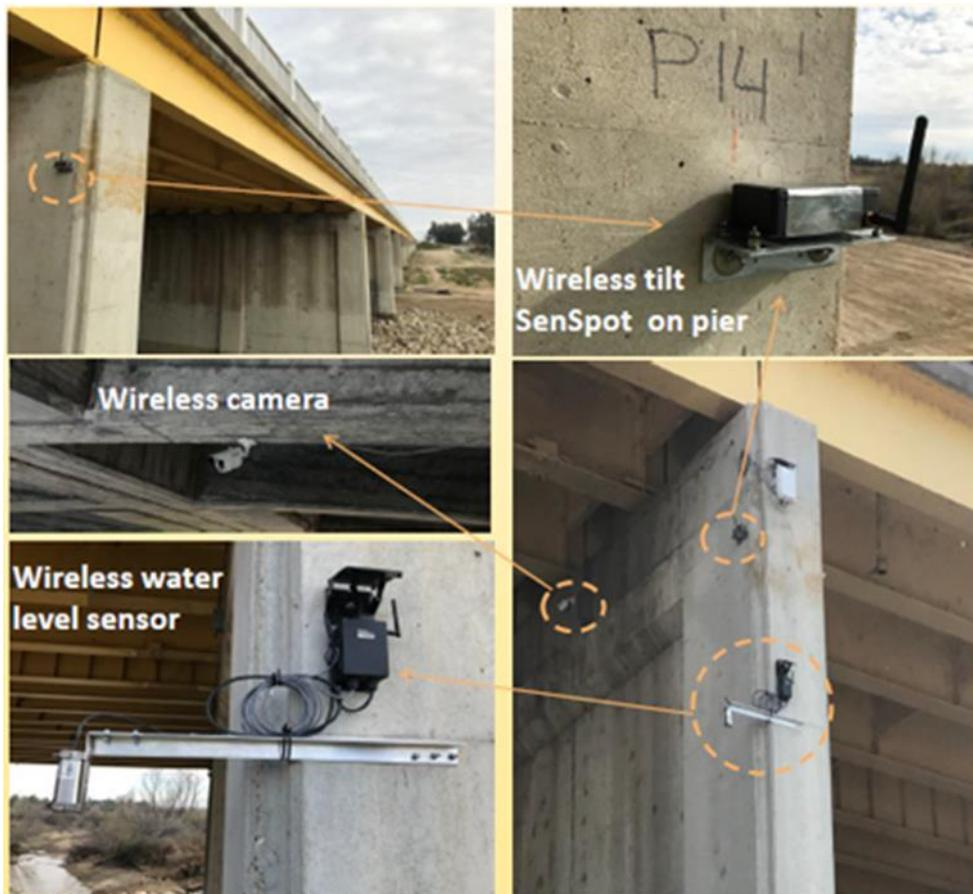
Resensys Wireless Tilt SenSpot™ sensor, Resensys Wireless Water Level SenSpot™ sensor and Wireless Solar Powered Camera on scour critical bridge
