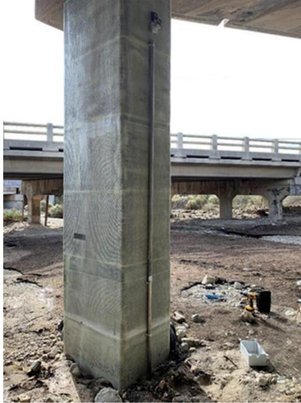
[Wireless Scour Probe SenSpot™ sensor](#) on pier of scour critical bridge to measure sediment level
